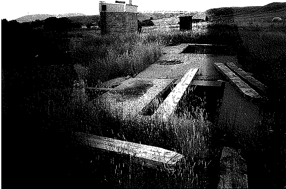
Looking north is truck off-loading area for grain hopper foreground, truck scale north, coal blockhouse northwest.
