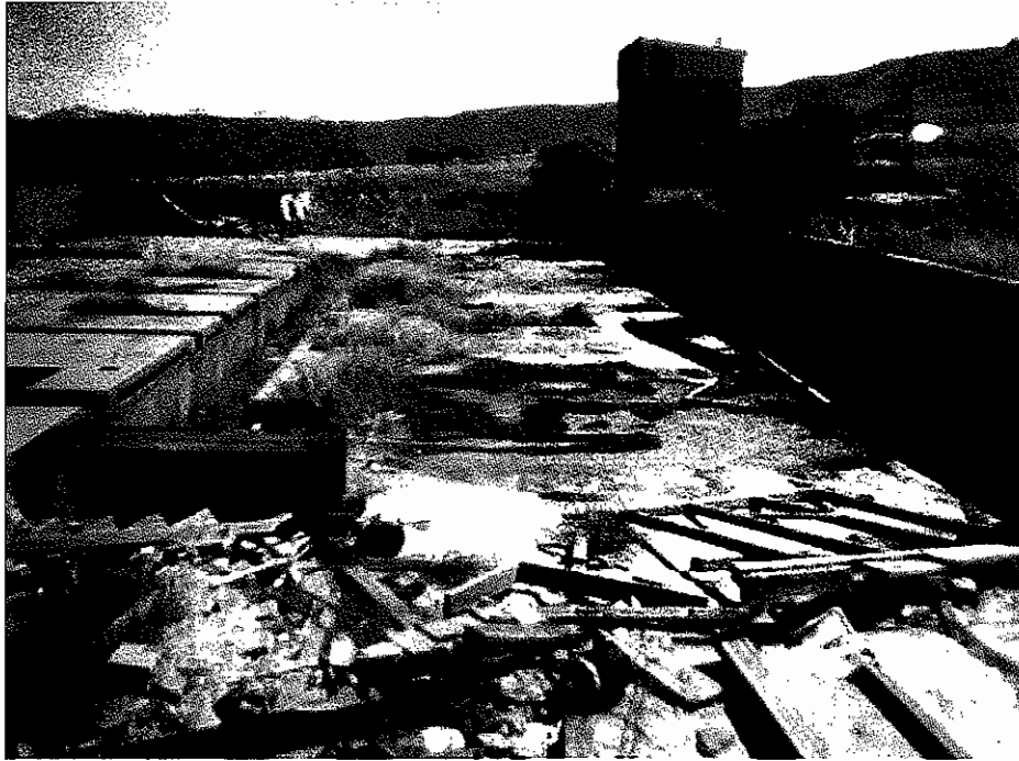
Main cement pad/building area looking north, trench on left Debris in foreground
