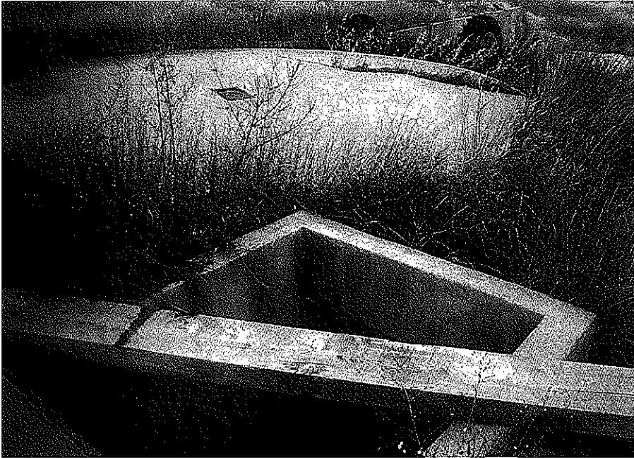
Underground cement silo for grain storage, approximately 15 feet deep, next to truck unloading hopper, cement pad for grain above ground steel silo in background; looking southwest
