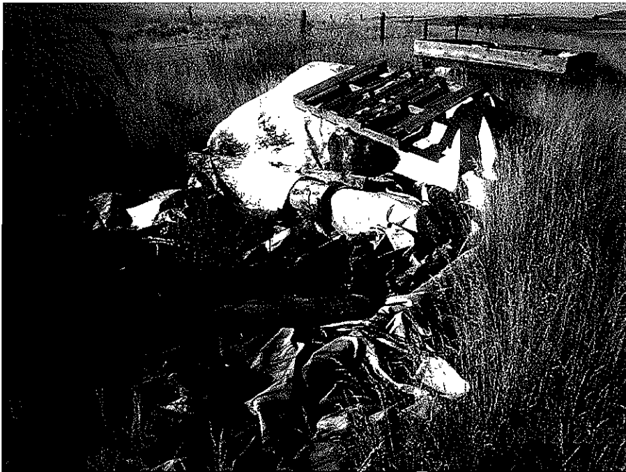
On-site storage of tarp covered wood in foreground, and trailer with asphalt shingles in the background along the east fence line; looking south
